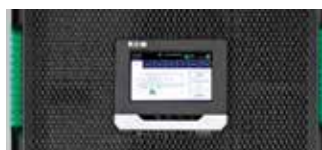
Green light bar showing healthy UPS
